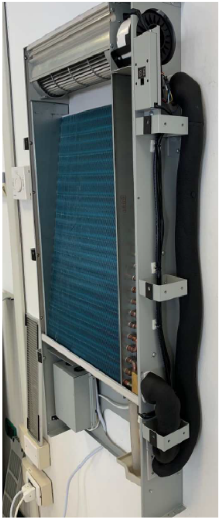
PUT INSULATION IN ALL THE EXTERNAL PIPE
